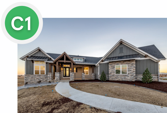
New Construction (Just Built)
