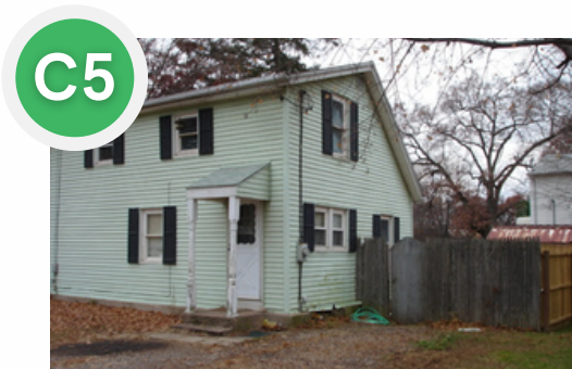
Fair (Major Repairs)
